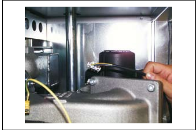
Fig.: Undo all electrical connections at the fan and the ignition transformer.
