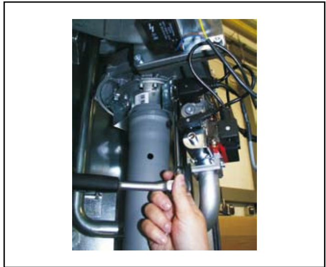
Fig.: Undo the screws between the fan and the mixing chamber.
